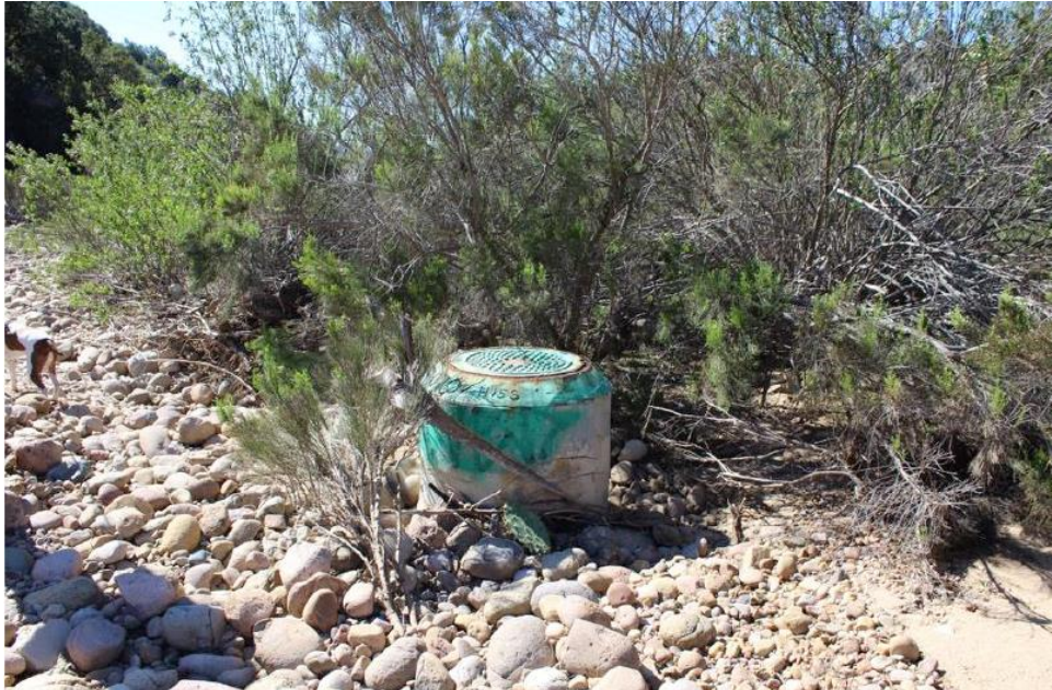
Example of utility access within Ruffin Canyon
