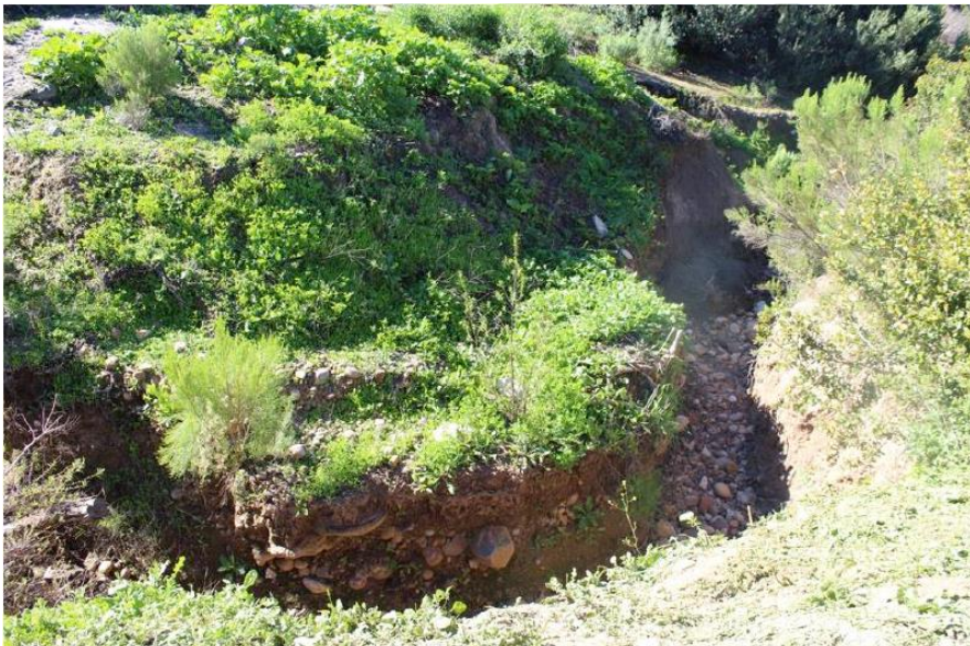
Incised channel created by unnatural erosion
