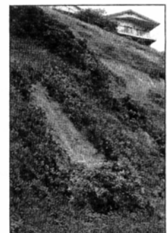
Ice plant gathers in a clump after recent rains washed away its hold on a hillside.
